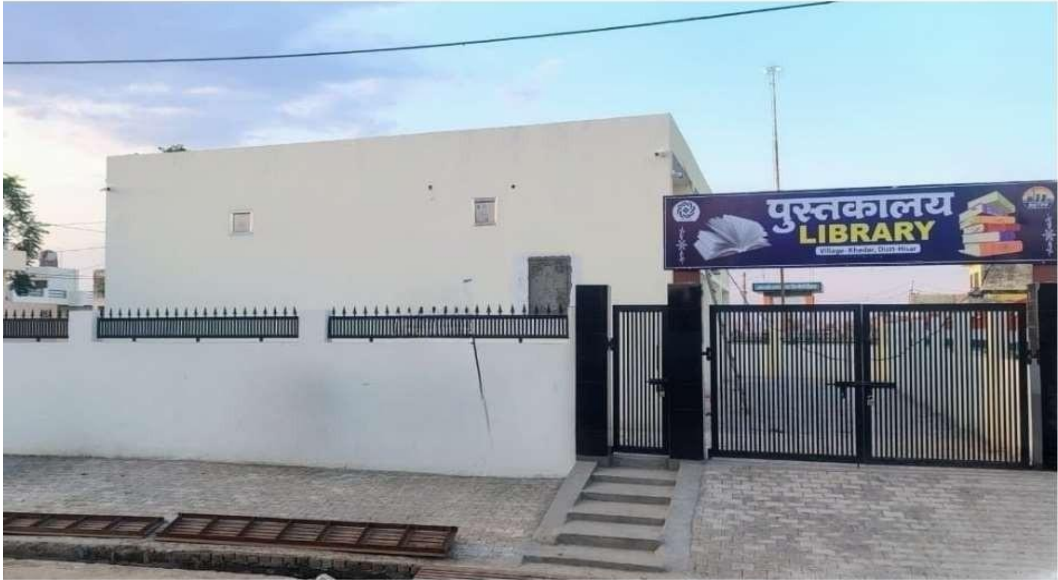
Photographs of library constructed under CSR initiative by RGTPP in Khedar village
