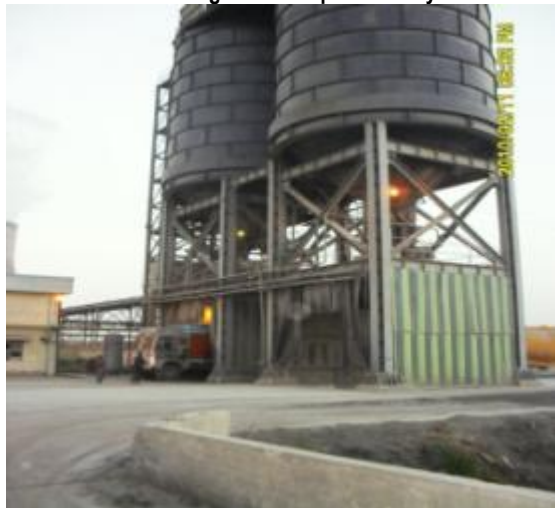
Fly-ash silo in Assan Khurd near Untla village
