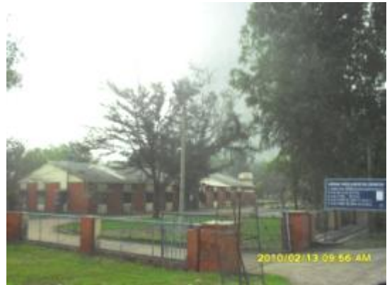
Photo B 1 – Administrative complex
