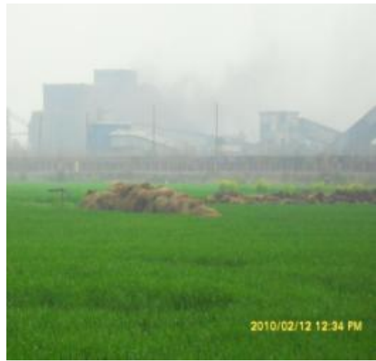
Photo A-4: Coal dust from the coal handling plant
