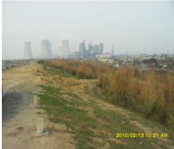
Natural vegetation atop the ash-dyke
